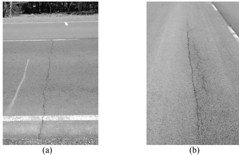
**Figure 14. (a) Transverse Crack in Section 2 and (b) Representative Wheel Path Crack in Section 3**
